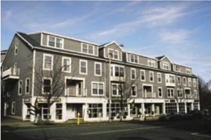
Mixed use development in Portsmouth, New Hampshire
